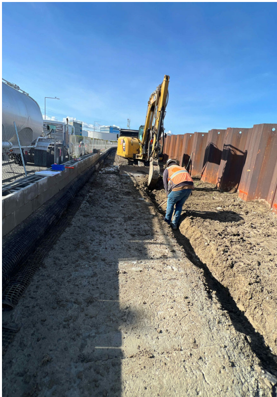
Levee retaining wall under construction
