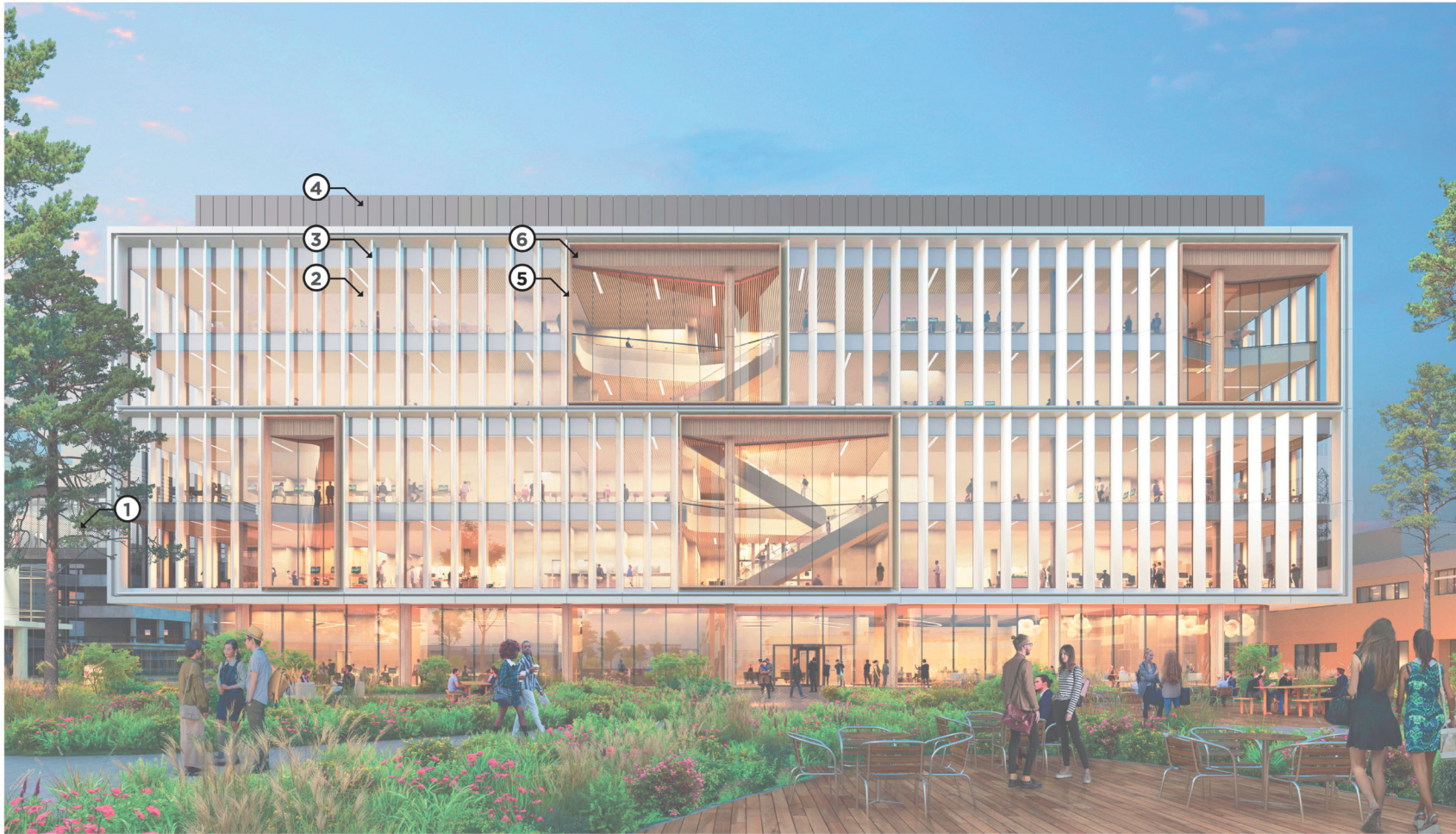
① INSULATED GLAZING UNIT WITH NEUTRAL LOW-E COATING ON CLEAR GLASS LITE WITH CERAMIC FRIT
